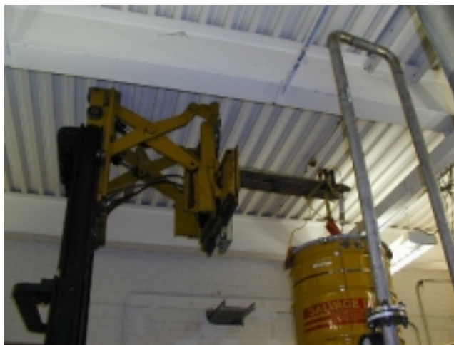
Figure 7. Lowering 85-gallon Overpack into the Pyrolyzer
